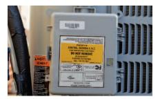
On hot summer days when electric use is at its peak, a Central Georgia EMC signal activates the Load Management Switch and temporarily cycles off your water heater during the peak demand period. Your central air conditioner compressor temporarily cycles off for 7  $\frac{1}{2}$  minutes each half-hour. The system's fan inside your
